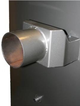
**TEE ADAPTOR FITTED AND SEALED. CONDENSATION CUP & ACCESS POINT AT THE BOTTOM**
